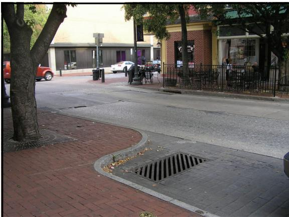
**YES:** Bulb-out used as a traffic calming device also reduces length of pedestrian crossing (West Chester Borough, PA).
